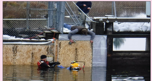
Divers and workers install Advantech sheathing.
